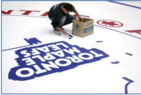
As suggested earlier in this guideline, some logos will create a natural heat transfer barrier resulting in warm spots on the ice that can cause a puck to slow as it passes over it. This same barrier have an impact on operating costs as the refrigeration system must run longer in order to maintain a quality ice surface. Using quality ice paint provides no such barrier while new textile logos have little to no barrier effect.
