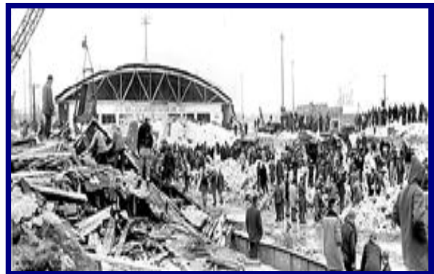
Listowel Arena Collapse-1959
