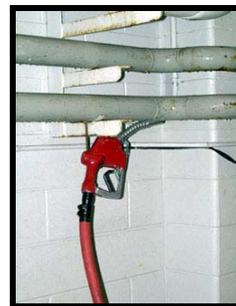
Figure 6: Water fill nozzle
