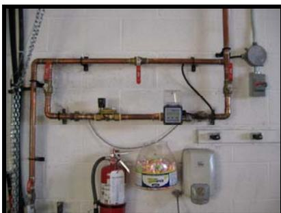
Figure 4: Computerized water valve system (Town of Milton)
